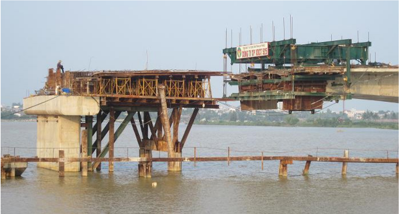
Road Project connecting Hoa Xuan Bridge and Hoa Quy ecological urban area Balanced cantilevered pre-stressed concrete structure
