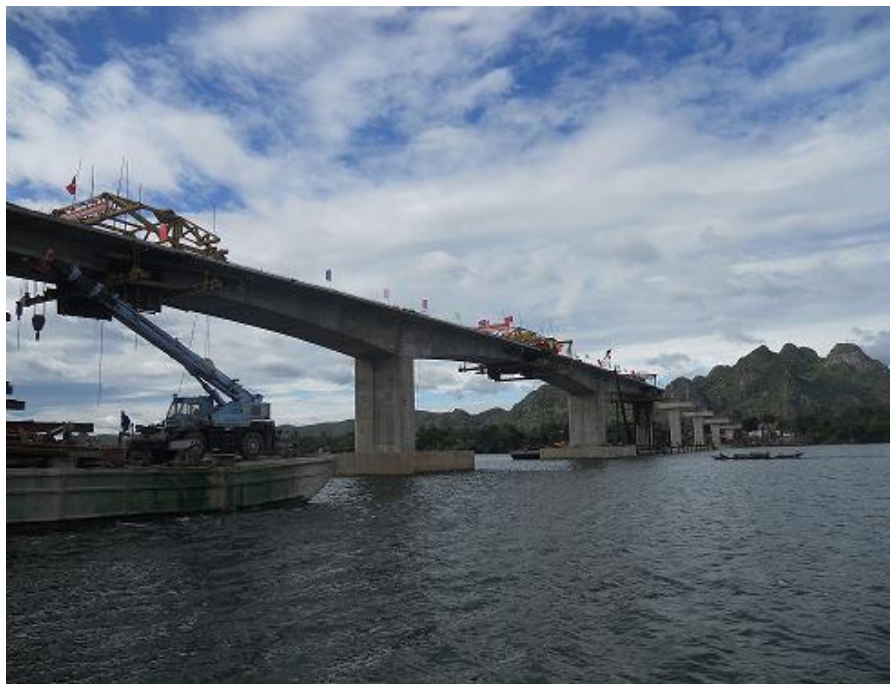
Bridge and road to Van Hoa commune, Tuyen Hoa District, Quang Binh Province Balanced cantilevered pre-stressed concrete structure
