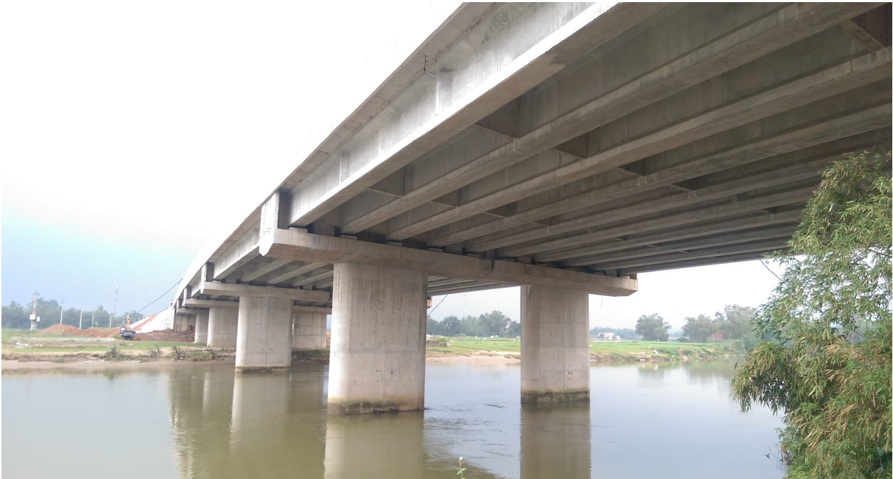
Package 01: Km0+00 Km8+00 LRB02 Bridge Km02+460.75 across Yen River – Danang City Pre-stressed concrete structure L=33m
