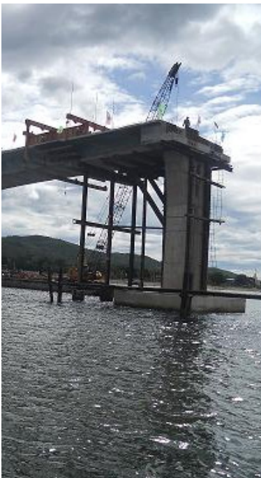
Bridge and road to Van Hoa commune, Tuyen Hoa District, Quang Binh Province Balanced cantilevered pre-stressed concrete structure
